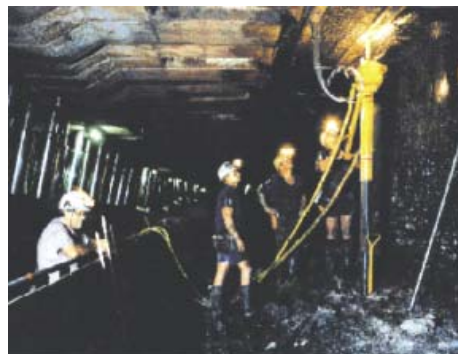
Underground Roof Bolting
